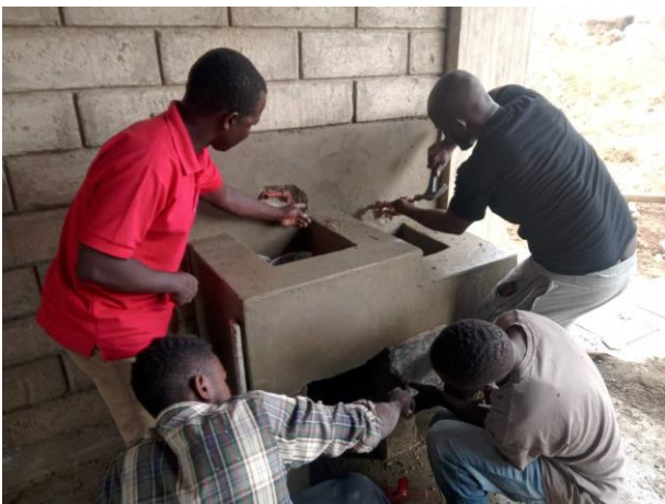
The tapstation is covered with Tarazzo plaster
