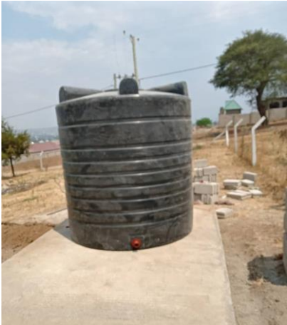
The first tank with 5000 litres is ready
