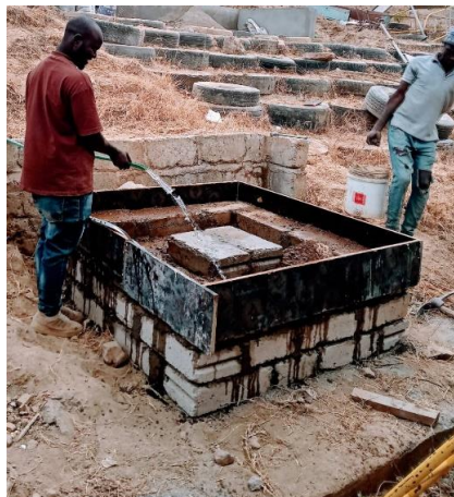
The new platform for the rainwater tank is being built
