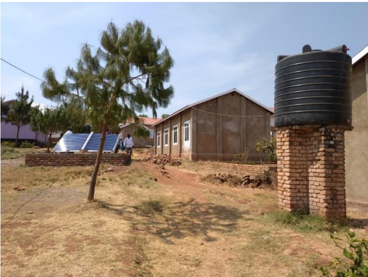
In the background: the platform after the first stage with one SoWaDis system. In the foreground: the central tank for safe drinking water with a capacity of 2000 litres.
