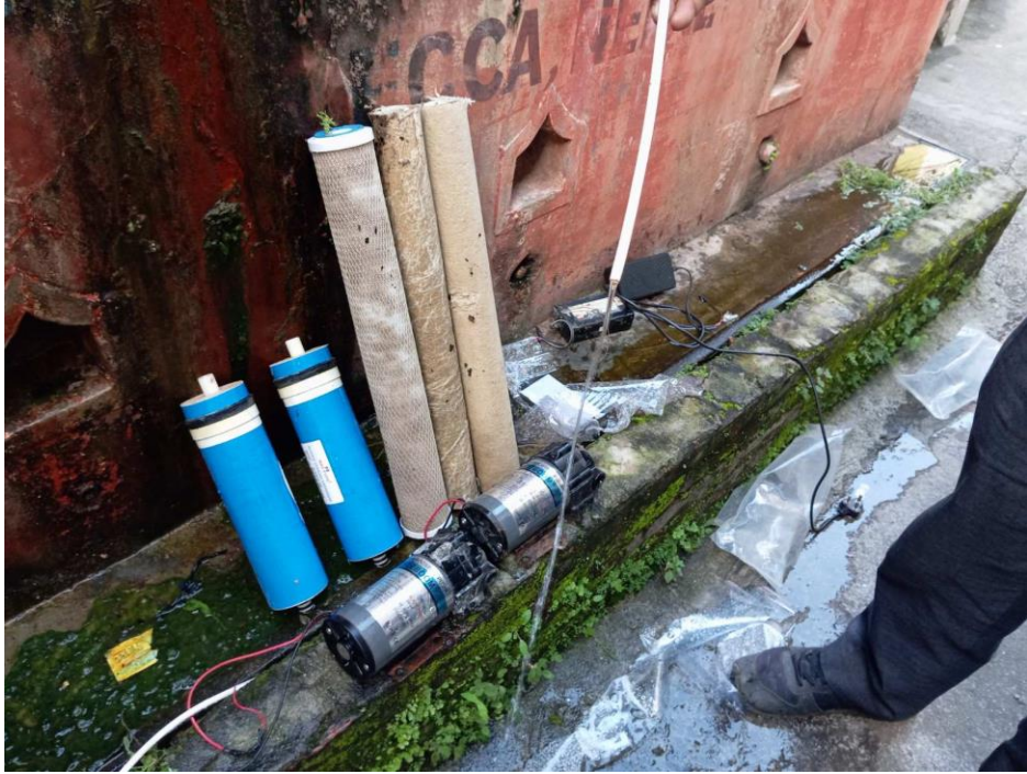
During maintenance work
